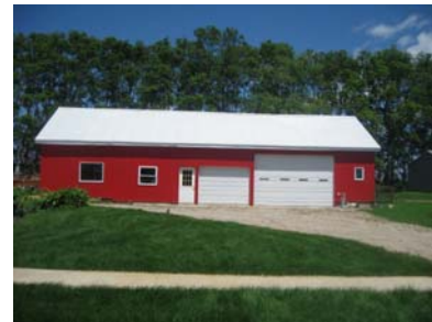
Machine shed/work shop
